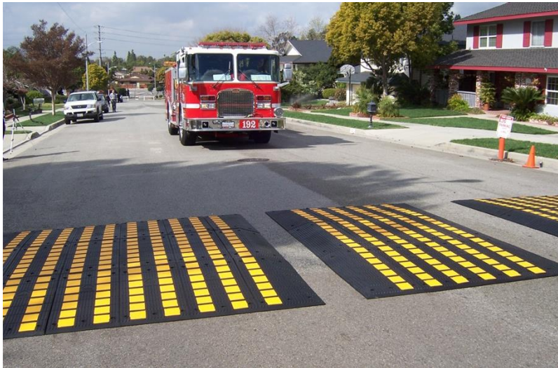
Example of speed cushion designed to allow large vehicles, such as emergency vehicles, to pass unimpeded
