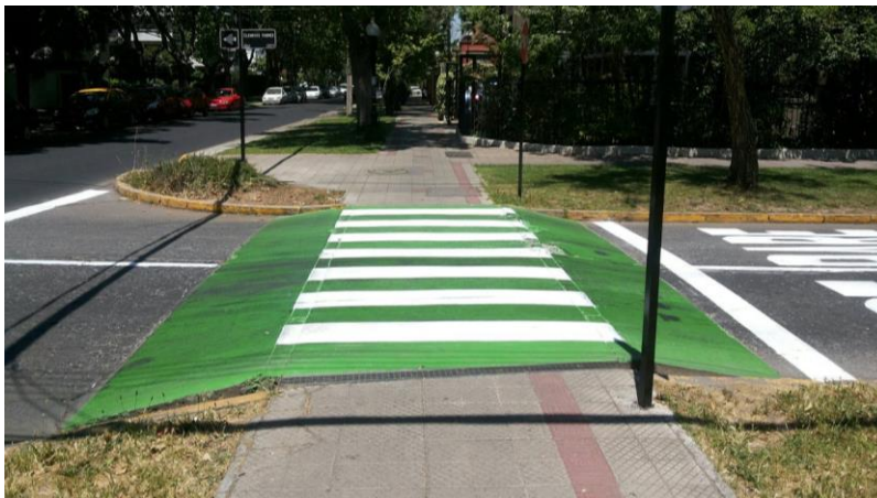
Example of a speed table with pedestrian crossing
