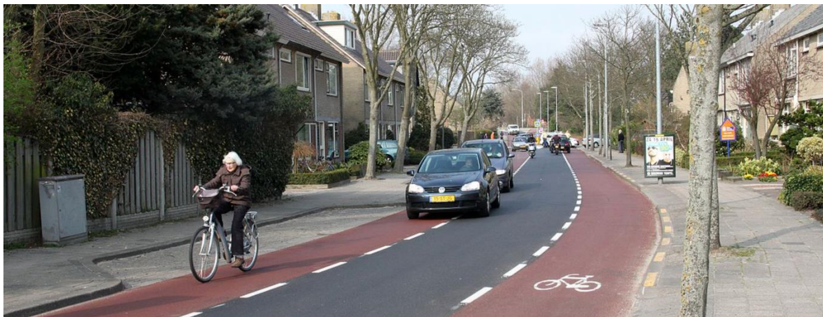
Figure 9 Example of a two-way local access road in The Netherlands, which uses bicycle lanes to visually reduce the width of the road 25
