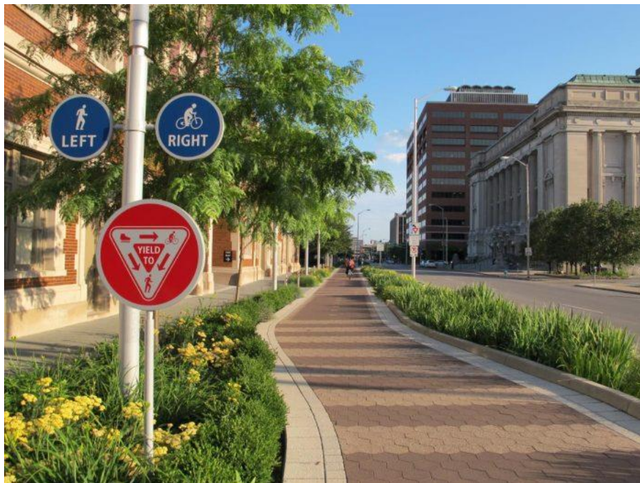
Figure 33 Example of garden beds and a bicycle lane acting as a ‘buffer’ to reduce crossing activity 58
