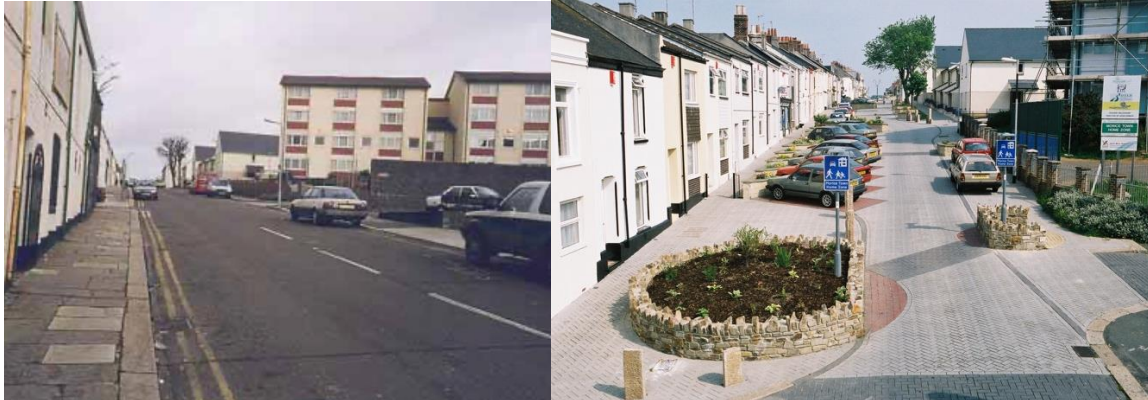
Figure 3 Before and after combined application of engineering traffic calming measures on a residential street (Charlotte Street, Morice Town, UK)
