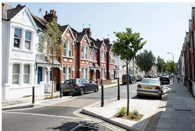
Figure 26 Example of a kerb buildout providing a safe informal crossing point in Hammersmith and Fulham, UK 48
