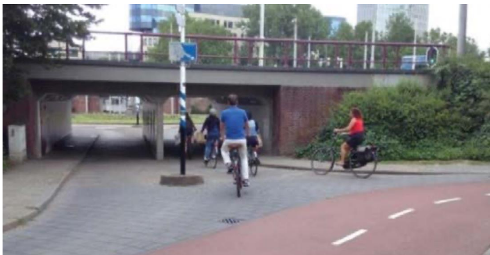
Figure 31 Example of a grade separated pedestrian and bicycle crossing in the Netherlands (DfT, 2020)
