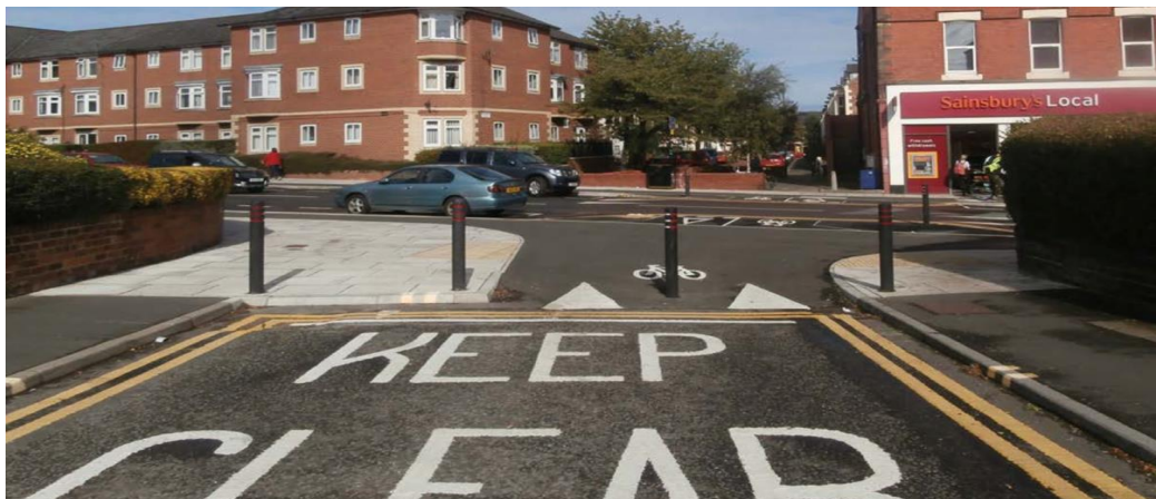
Figure 23 Example of a full intersection closure designed to allow free passage by bicyclists and pedestrians (DfT, 2020)
