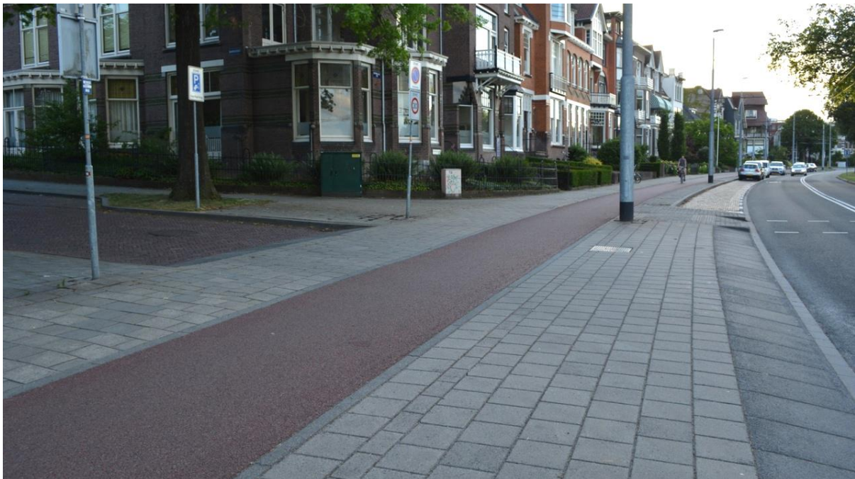
Figure 28 Example of a flush crossing and bicycle path across a side street entry in The Netherlands 52
